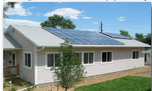
Photo courtesy DOE/NREL - The panels at upper right are for hot water, the ones on the left make electricity. (Photo 7)
