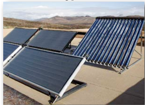
Photo The Radiant Floor Company Two types of solar hot water heating panels (Photo 5)
