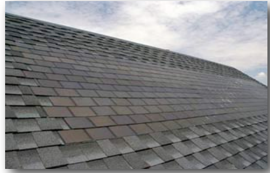
Photo courtesy DOE/NREL - 'Solar Shingles' may be nearly invisible on the roof. (Photo 8)
